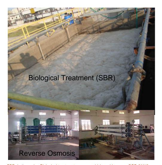
SBR is the only Biological treatment process which could remove COD &NH3 from Pharma or Pesticide effluents.
